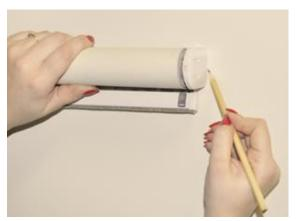
1. Place the cornice firmly horizontally on the wall and make markings on both sides of the cornice where you will attach the brackets.
