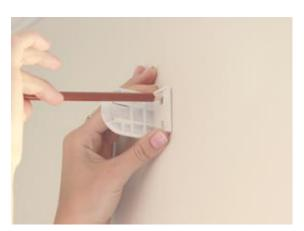
2. Place the brackets on the markings and mark points in the mounting holes, where the mounting brackets will be placed.
