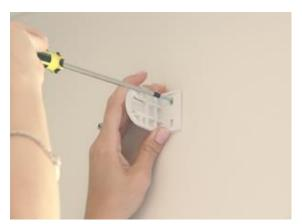
3. Screw the brackets to the wall through the mounting holes.
