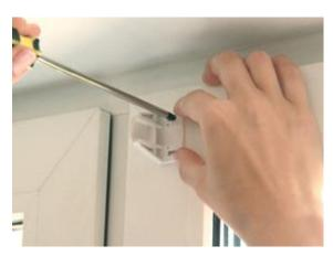
2. Screw the blind fasteners to the window frame.
