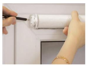
1. Attach the cornice to the window frame and mark both sides.
