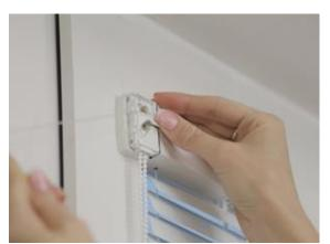
8. Stretch the string up and lock it with the blind covers. Cut off the excess part of the string.
