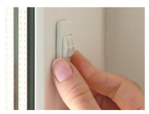
10. Screw the chain holder to the window frame at the desired height. Attach the control chain.
