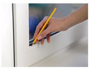
5. Mark the distance on the bottom bead of the window with a pencil to attach the string holder. The string must be at right angles.
