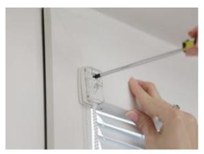
4. Screw the blind mechanism through the mounting holes.
