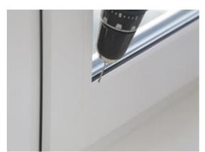
6. Drill hole for attaching the holder.
