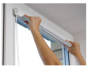
3. To determine the fastening points, place the cornice horizontally between the side beads of the window and mark the place for screwing.
