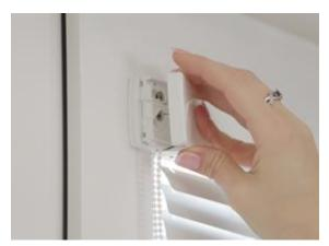
9. Put the top covers on the mechanism.
