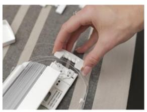
2. If necessary, install the spacers so that the slats can move freely without touching the glass.
